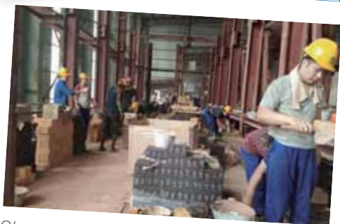
Glass factory construction site: building northern regenerative chamber
